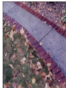
New Brick Boarder
